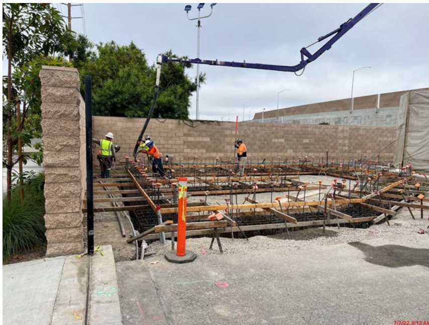
Figure 25. Construction of the Southwest Storage Building at the MWRF
