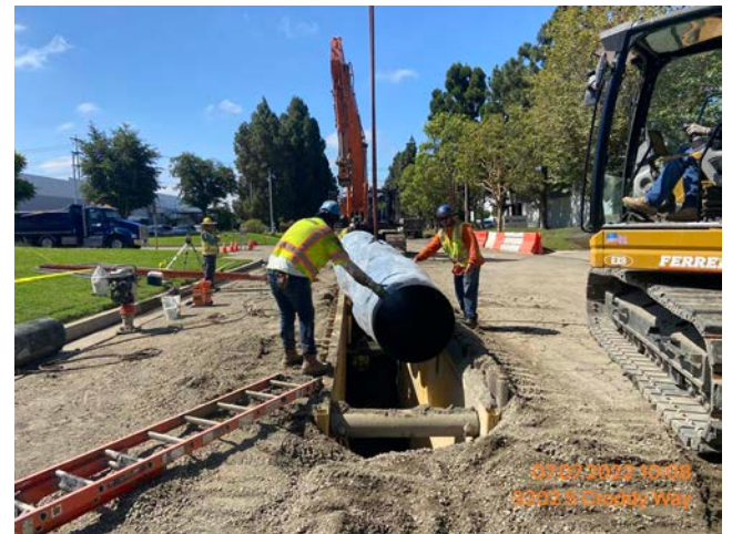
Figure 6. 30-inch Pipeline on Croddy Way
