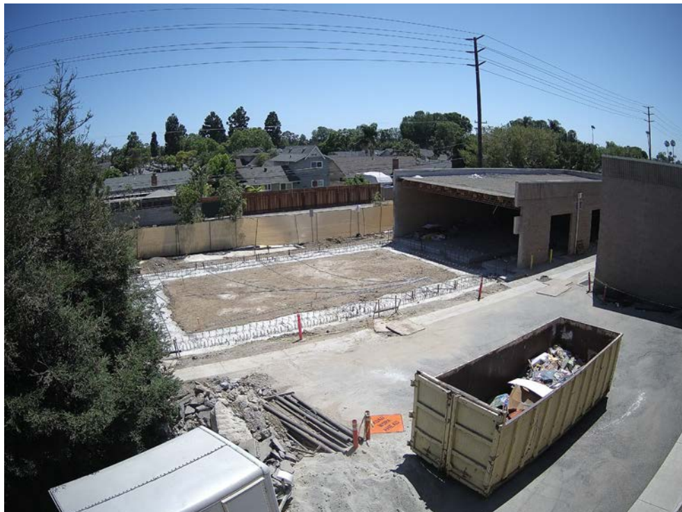
Figure 22. Administration Building Demolition
