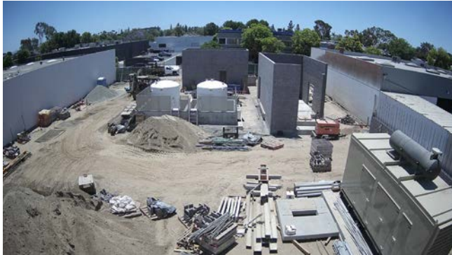
Figure 3. Well No. 12 Building Construction
