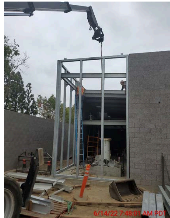
Figure 2. Well No. 14 Well Building
