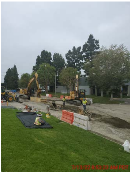
Figure 5. 30-inch Pipeline on Croddy Way
