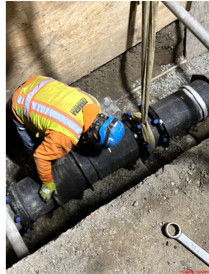
Figure 6. Connection to Mesa Water Distribution System
