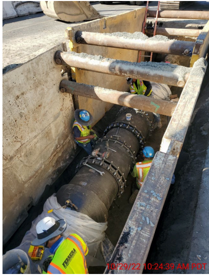
Figure 5. 30-inch Pipeline on MacArthur
