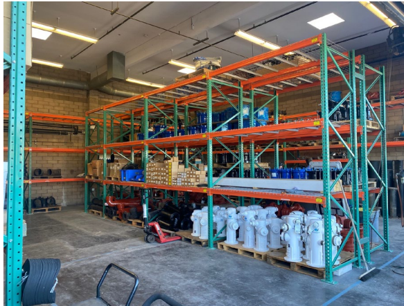
Figure 24. Garage Storage Project Photo
