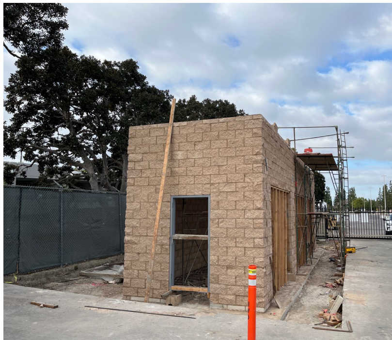
Figure 25. Construction of the Well Parts Storage Building at Well No. 7
