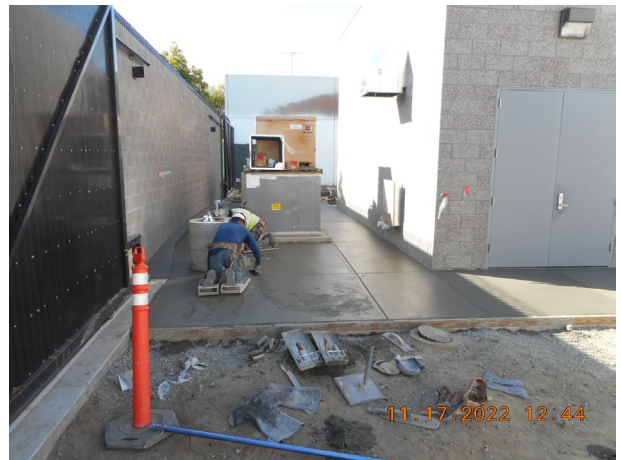
Figure 2. Well No. 12 Site Concrete
