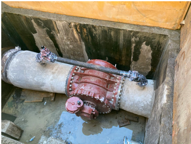
Figure 14. Vault Rehabilitation and Abandonment Project Bonita Creek Vault Installation
