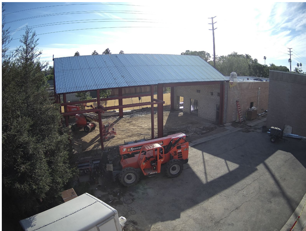
Figure 22. Mesa Water Education Center Steel Framing
