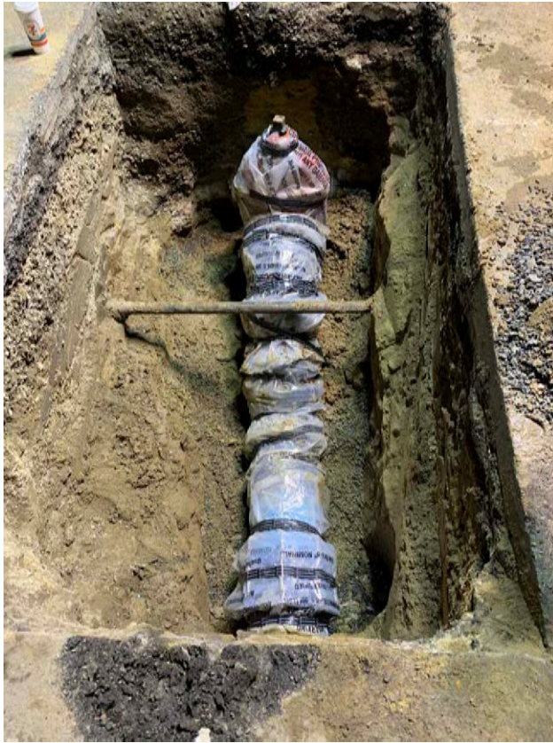
Figure 9. Mainline Valve Replacement
