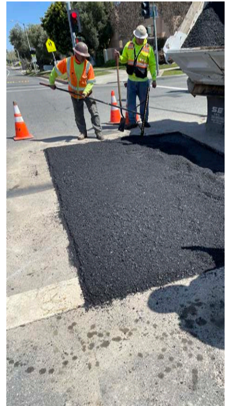
Figure 10. AC Pavement Repair
