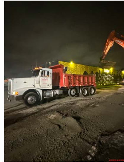
Figure 6. 16-inch Pipeline on Chandler Avenue
