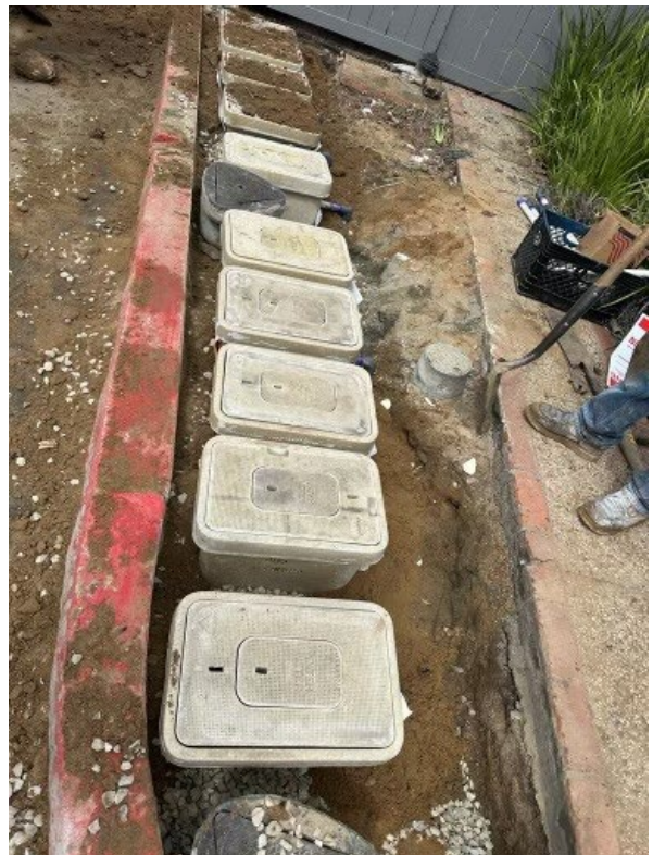
Figure 13. Meter Box Installation
