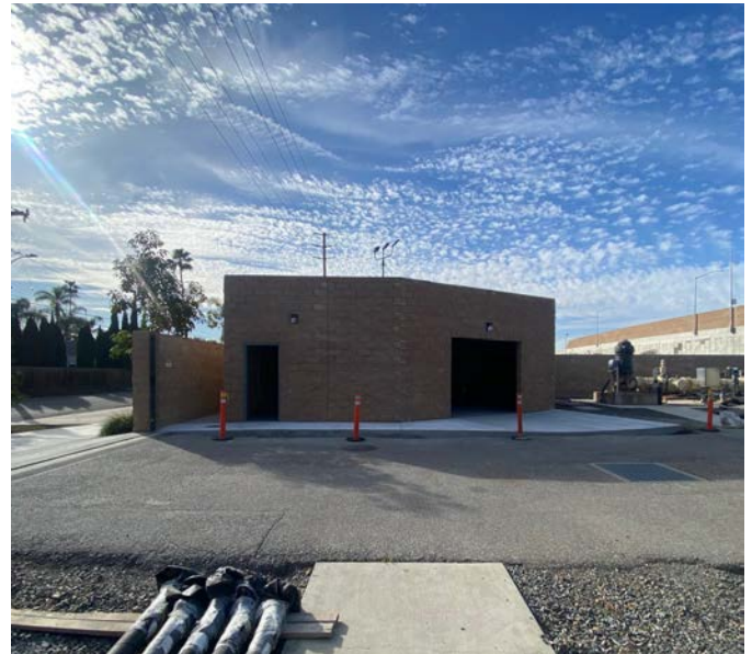
Figure 21. Southwest Storage Building
