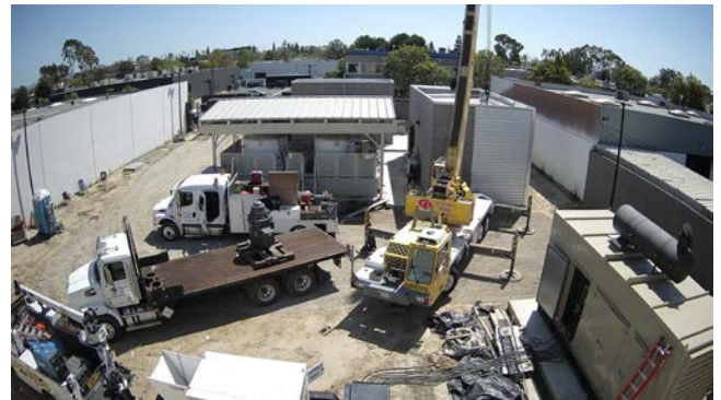
Figure 4. Well No. 12 Well Pump Installation
