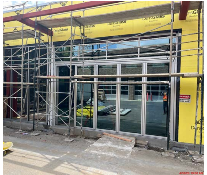
Figure 16. Folding Door Installation
