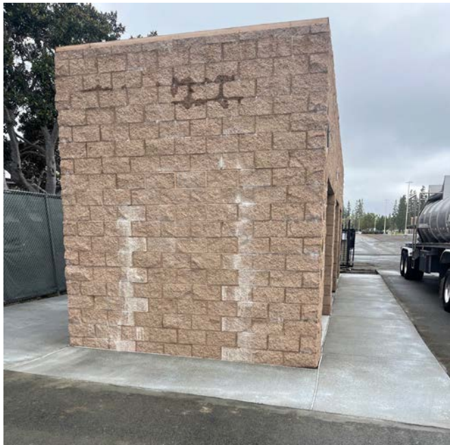
Figure 20. Well Parts Storage Building
