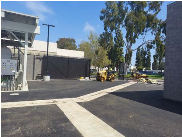
Figure 3. Well No. 14 AC Pavement
