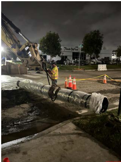
Figure 5. 16-inch Pipeline on Chandler Avenue
