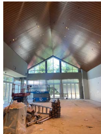
Figure 6. Education Room Ceiling Installation
