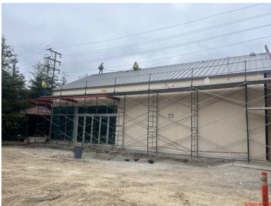
Figure 5. Education Center Roof Installation
