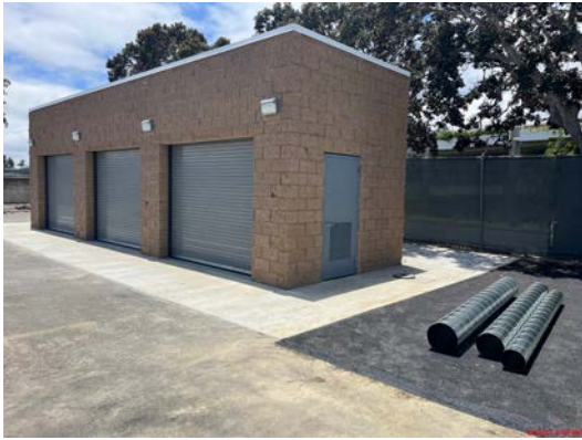
Figure 8. Well Parts Storage Building
