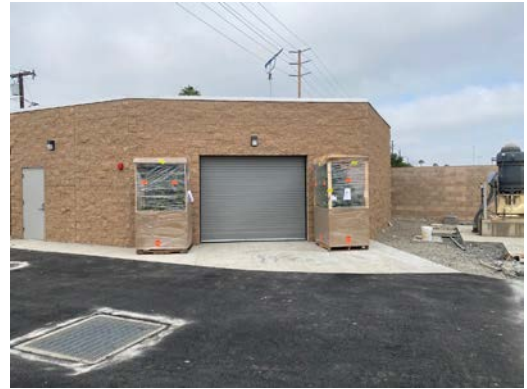
Figure 9. Southwest Storage Building
