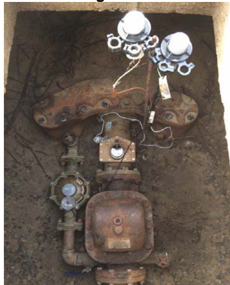
Figure 9 – Converted TR Universal CE Meter Vault
