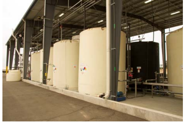
Figure 3-7. Sample High-Density Crosslinked Polyethylene (XLPE) Tank
