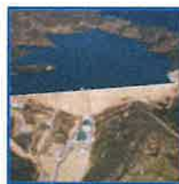
Olivenhain Dam & Reservoir $198 million
