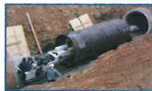
Pipeline Relining $493 million
