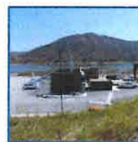
Lake Hodges Hydroelectric and Pump Station Facility $208 million
