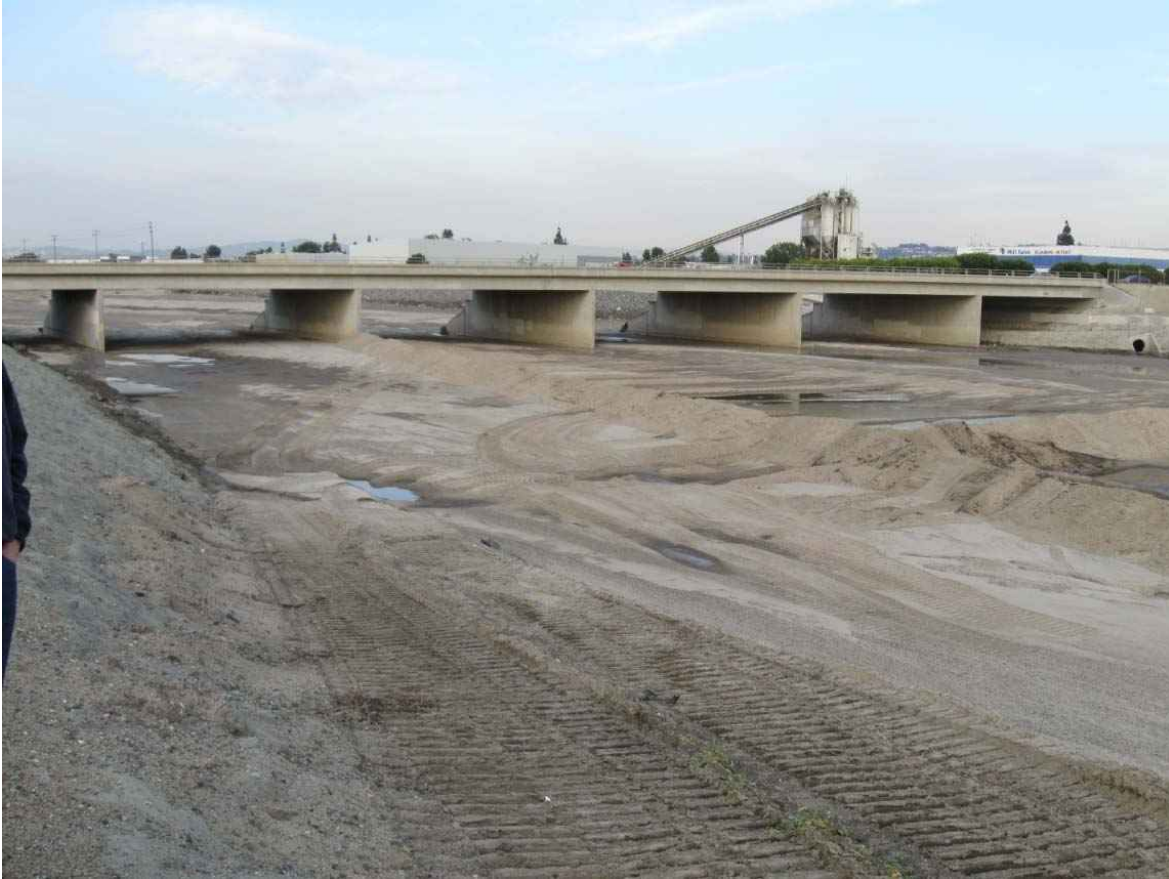
Figure 14-2: Santa Ana River, looking upstream in the vicinity of Ball Road. Here the river, with side levees and a soft bottom, is typically dry during non-storm conditions.
