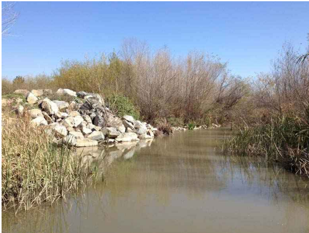
Figure 14-1: Santa Ana River, downstream of Prado Dam
