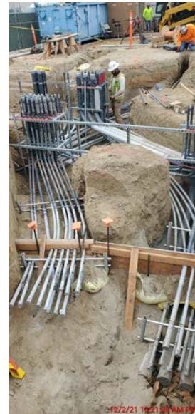
Figure 2. Electrical Ductbank Installation
