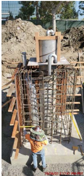
Figure 1. Concrete Well Pedestal Installation
