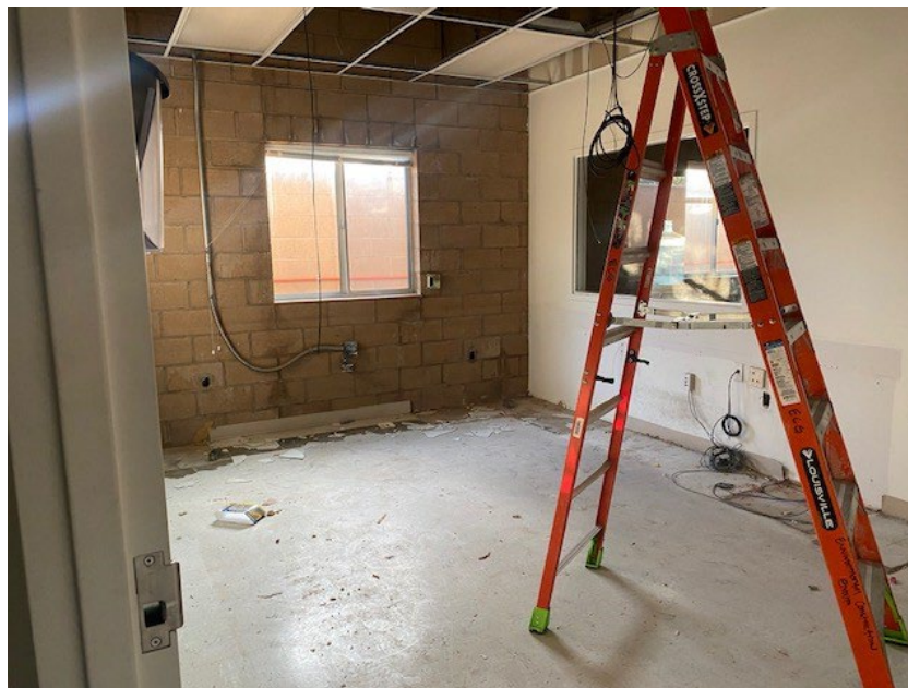
Figure 22. Demolition of Existing SCADA Control Room
