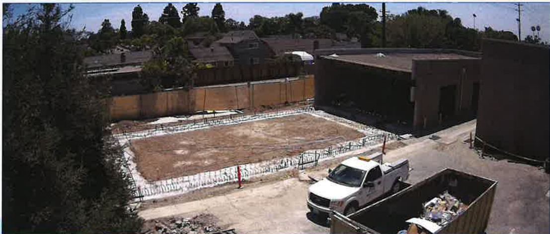
MWRF Administration Building
