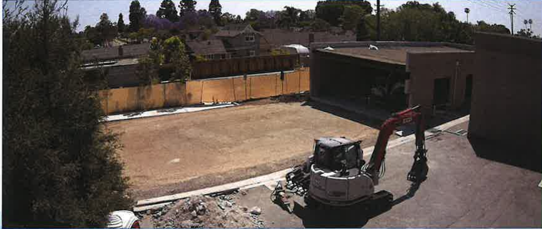
MWRF Administration Building
