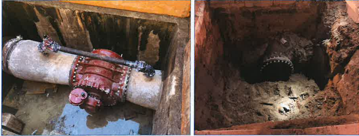
Vault Rehabilitation and Abandonment Project
