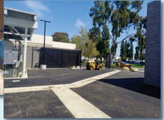
Croddy Well Site July 2023
